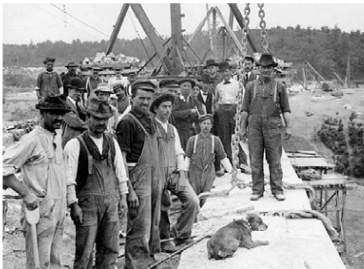
"The Braccianti" take time to pose at the top of the Wachusett Dam while still under construction, around 1905.
