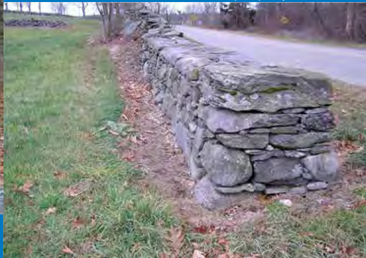
This nicely constructed estate wall, below, shows how a skilled mason took the time to give careful attention to form and fit of the stones as a statement to the landowner's prosperity.
