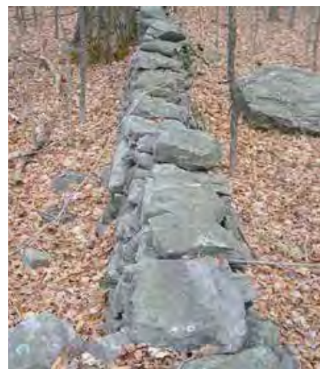
The more carefully constructed "stacked wall" was built to endure the ravages if time, and very likely used to de-mark a property boundary.
