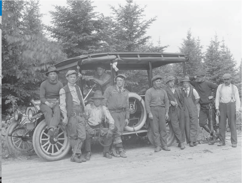
Above right: This 1918 image shows 10 electrical transmission laborers working on the Wachusett to Sudbury power lines, posed around a contractor's truck.
