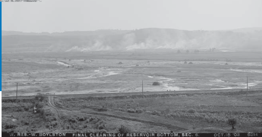
W. RES.-W. BOYLSTON FINAL CLEANING OF RESERVOIR BOTTOM, SEC. 6.
