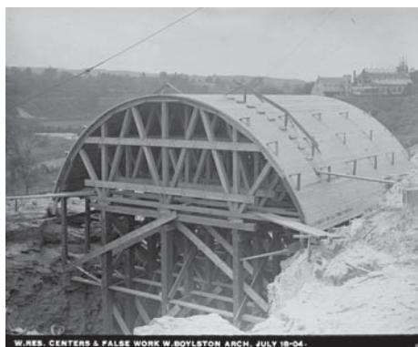
W.RES. CENTERS & FALSE WORK W.BOYLSTON ARCH. JULY 18-04.
