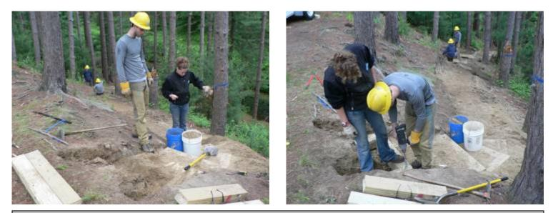
Steps along the steeepest portion of the trail are cut into the bank, placed and secured (above). The upper terraces are put into place, leveled secured with pipe pins on the corners and stabilized from beneath with rocks and soil (below).
