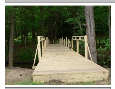
Top railings were added to meet code (above), and then finished off with balusters and caps (above right). Soil was added at either end to make the approach to the bridge level. Wood chips were also added for landscaping and to reduce erosion problems. The height of the bridge above the river allows unimpeded access for anglers who patrol this section of the river in search of trout (right).
