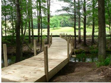
The original arch trusses were used to support the new joists. Posts for hand rails were added at intervals across the structure.
