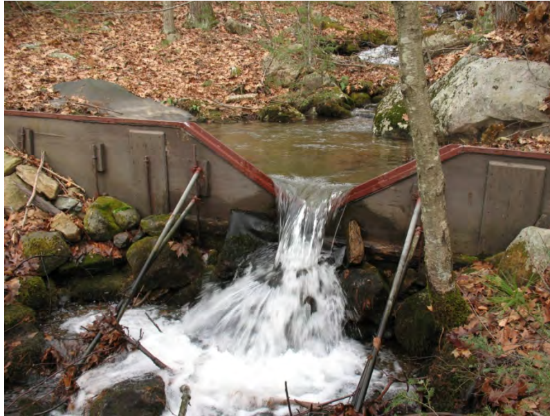
Figure 4: Shays Brook downstream weir December 2011
