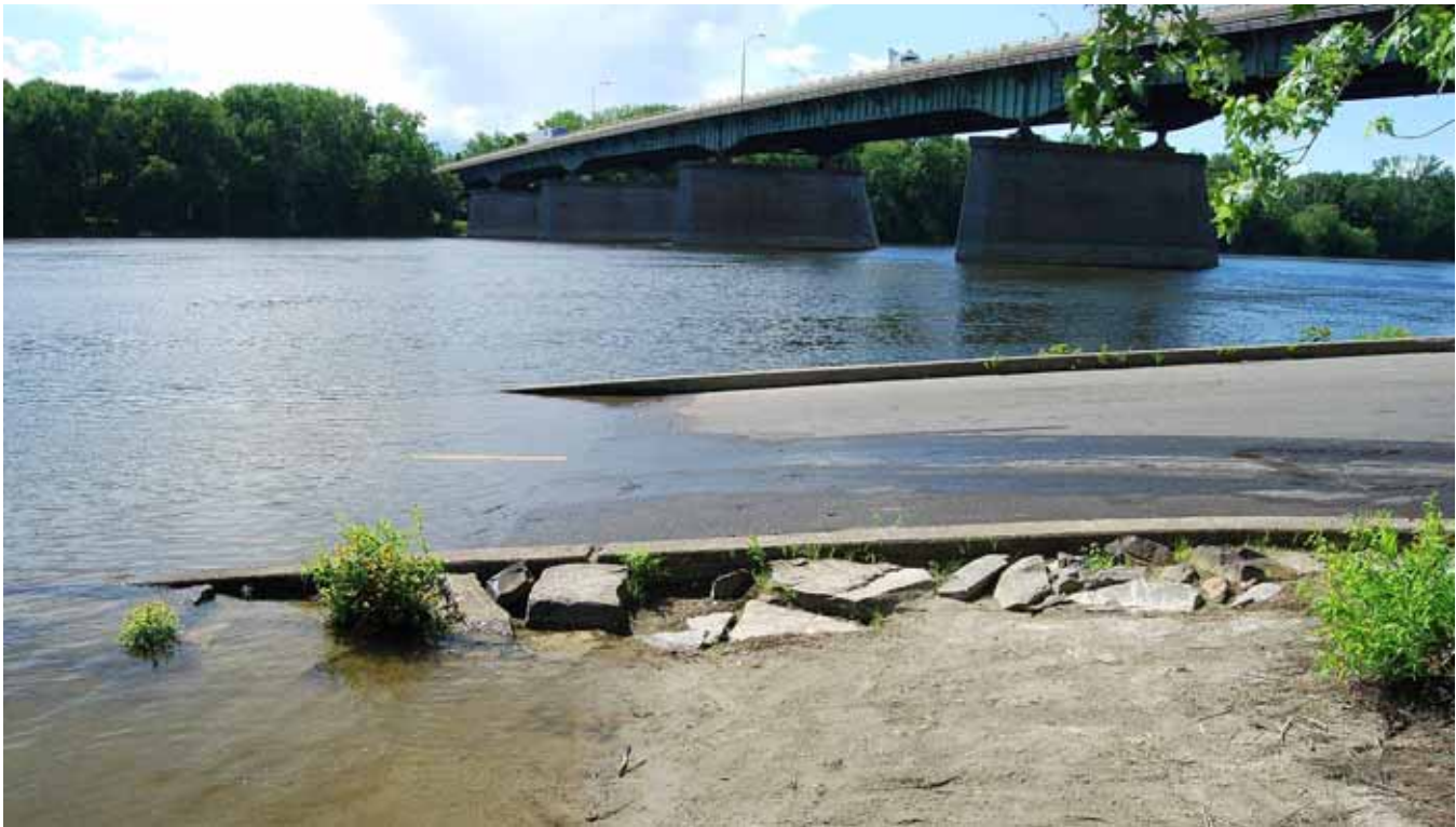
OFBA ramps, such as this one in Chicopee, were targeted for surveys in the Connecticut River.
