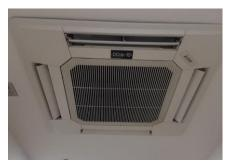
ASHPs use a refrigerant loop to extract and move heat between spaces. Systems can provide both heating AND cooling.
