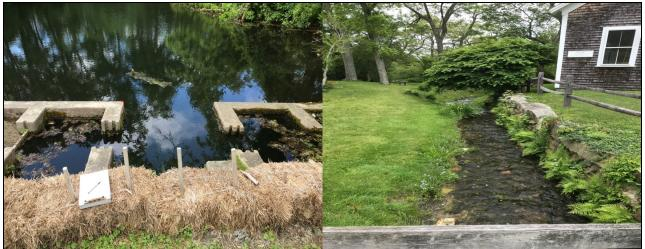
Figure 3: Concrete dam/spillway structures controlling water levels on the upstream side of site S4.
