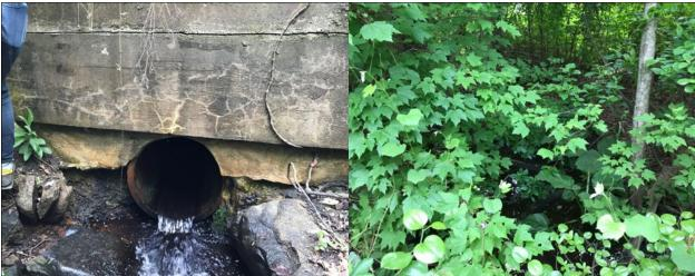
Figure 34: The downstream structure of site B3 is a small metal culvert that is slightly perched during typical low flow conditions.
