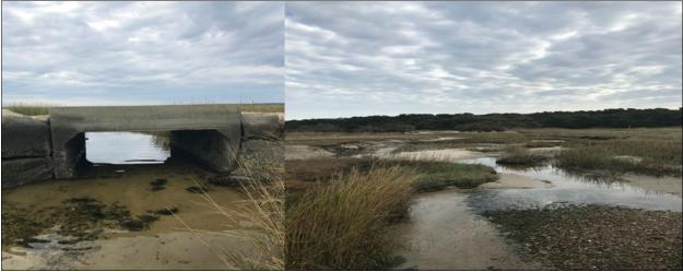
Figure 41: The upstream side of site B23. The structure is in good condition and rock retaining walls have been put in place around the opening to limit erosion and washout of the trail.
