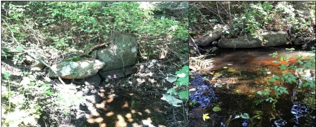
Figure 69: Field observers were unable to identify what kind of structure was covered by the stone at site Y4, shown here on the upstream side. Due to the small opening beneath the stone, debris has accumulated at the crossing.
