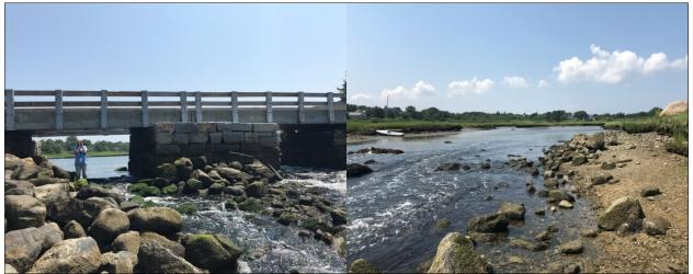
Figure 54: A stone support splits the bridge opening into two passageways for water flow and the bridge is heavily armored with large rocks on both sides at site Y1.
