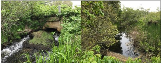
Figure 37: A large mass of peat is partially blocking flow on the downstream side of site B7, most likely rafted up during the blizzard in January 2018 or the northeasters in March 2018.
