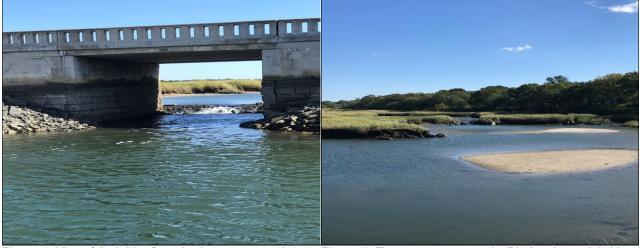
Figure 45: View of the bridge from the downstream marina. Notice the perch created by the rip rap located on the upstream side of site B25.
