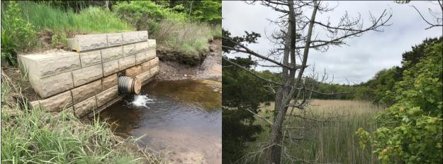
Figure 12: The flap gate on the downstream side of site S5 presents a tidal restriction, shown here at low tide.
