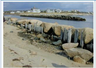
Photograph 2.1. Coastal beach with jetty. Although there is a jetty on this beach, the sand is still able to respond to wave/water activity by shifting and changing form as seen from the sand that is being eroded from behind the jetty. The amount of sediment exchange between the beach on the left and right of the rocks, however, has been restricted by the jetty.
