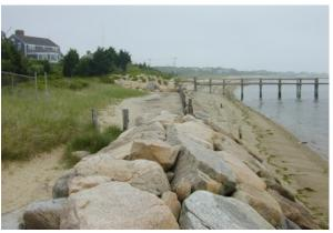
Photograph 1.9. Coastal dune with coastal engineering structures. Foreground: coastal dune landward of rock revetment. Background: coastal dune and beach landward of a deteriorated bulkhead.
