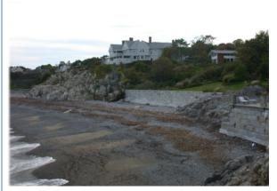
Photograph 2.15. Coastal bank serving as a vertical buffer. This rocky coastal bank and seawall act as a vertical buffer to protect inland areas. The base flood elevation is below the top of the coastal bank (top of wall) and erosion of materials above the wall (or rocky bank) has not occurred. This bank therefore does not serve as a sediment source due to its inability to erode by wave action and does function as a vertical buffer withstanding erosion from waves, wind, and rain.
