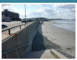
Photograph 2.3. Coastal beach with seawall. In spite of the seawall, this coastal beach is able to both shift and change form in response to waves and tides and to transport sediment along the shore. There is no longer a dune to serve as a reservoir of sediment for the beach.
