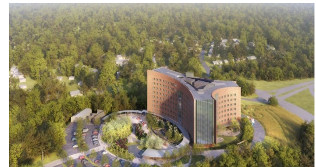
Holyoke Veterans' Home – under construction
